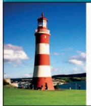
In 1756, John Smeaton built a stone lighthouse off the U.K. coast. He noted that unlike ordinary mortars of limestone and sand, those that also had a high proportion of clay became harder in water and could withstand the pounding of the waves. Shown here is the lighthouse, which was rebuilt on land as a memorial.
